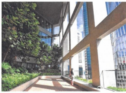
CapitaGreen's energy-saving features include a red flower-like wind scoop (above) at the top of the 40-storey building and a double-skin facade (left) to reduce heat gain. PHOTOS: CAPITALAND, JASMINE CHOONG
