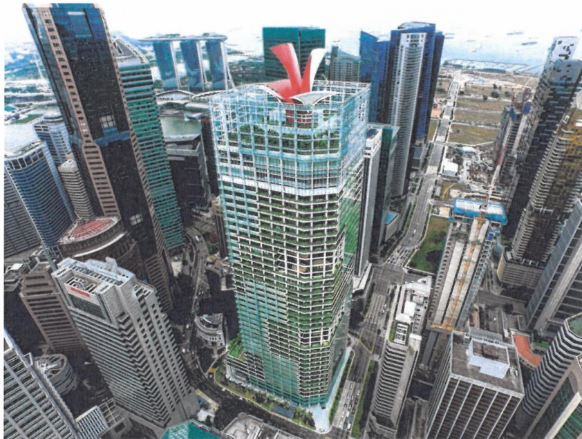
CapitaGreen's energy-saving features include a red flower-like wind scoop (above) at the top of the 40-storey building and a double-skin facade (left) to reduce heat gain. PHOTOS: CAPITALAND, JASMINE CHOONG
