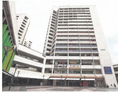
Mr Derek Teo (far left), leader of special verticals and key account management at Johnson Controls, at the chiller plant in Joo Chiat Complex (left). The firm retrofitted the old building with a state-of-the-art chiller system, and helped save close to 1.2 million kWh and $250,000 in utility costs. PHOTOS: KHALID BABA, LIANHE WANBAO FILE
