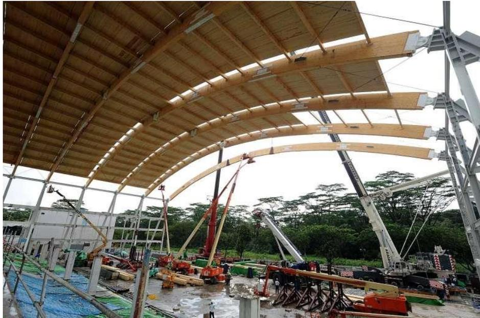
NTU's new sports hall uses glued laminated timber, or glulam, for its roof. It is lighter than steel, needs 60 times less energy to produce, and was assembled in less than a month. ST PHOTO: AZMI ATHNI
