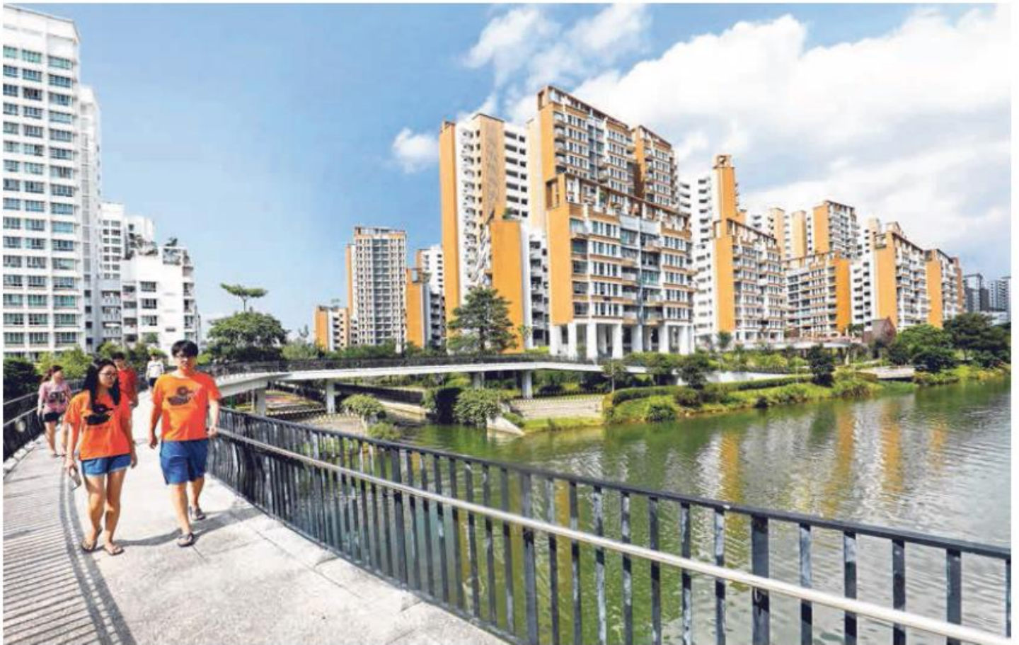
The Waterway View project in Punggol harks back to the estate's beginnings as a "kelong" or fishing village with features such as a textured facade that mimics wood for the 10 blocks, which are also staggered to allow as many of their residents as possible to enjoy the view of the waterway. PHOTO: LIANHE ZAOBAO
