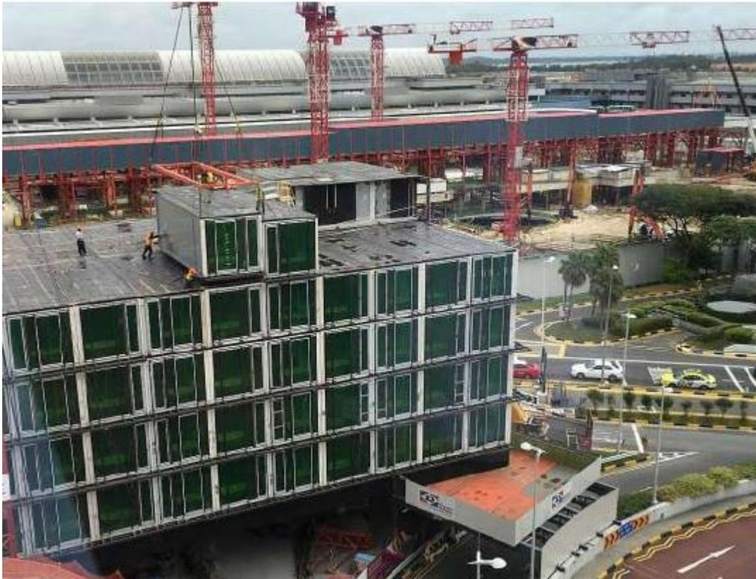
Crowne Plaza Changi Airport's new 10-storey extension being built using the more productive Prefabricated Prefinished Volumetric Construction technology. PHOTO: CROWNE PLAZA CHANGI AIRPORT
