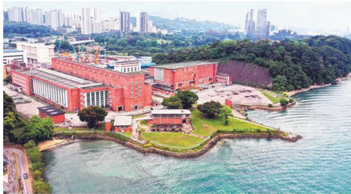
The Pasir Panjang Power District (left) is home to two red-brick main station buildings, round oil tanks and ancillary buildings, and it will be one of the first few sites to be developed along the Greater Southern Waterfront. PHOTO: URBAN REDEVELOPMENT AUTHORITY
