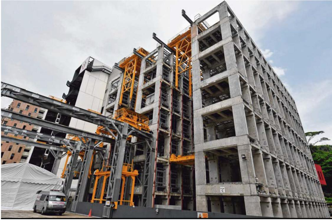
**An automated precast storage facility at the integrated construction and prefabrication hub, Greyform Building, in Kaki Bukit. Such hubs optimise land use and require less time and fewer workers to build. ST PHOTOS: JOYCE FANG**
