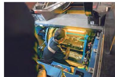
Technician Loh Fah Leong wiping excess oil from the inside of the escalator pit at Fortune Centre after completing the inspection. The 51-year-old has 23 years of experience in the repair and upkeep of lifts and escalators.
