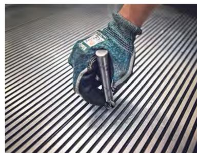
A special lifting device being used to open the floor plate bolt of an escalator at Republic Plaza. This is the first step that technicians must take in order to gain access to the escalator pit, where the servicing work will take place.
