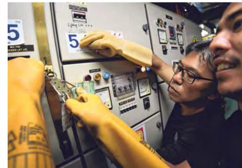
Locking the circuit breaker in "off" mode is a must before service foreman Hou Heng Choon (left) and technician Mohd Iskandar can start work in the lift motor room at Republic Plaza. This step ensures the system does not get switched on while they are working on high-voltage components.
