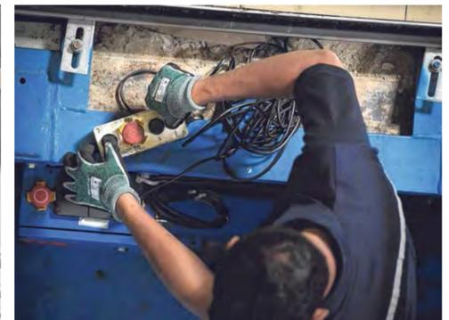
An escalator technician using an inspection device to move the steps in the desired direction. As a safety feature, he must press the green "Start" button (at his left) together with an "Up" or "Down" button to make the steps move.
