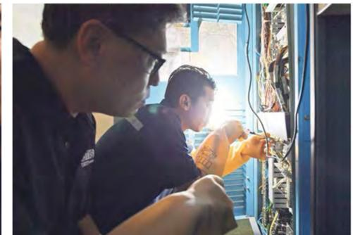
The two men start their maintenance routine in the lift motor room by checking the condition of the lift machinery and ropes. The procedure includes thoroughly testing the high-voltage circuits of the lift controller – the "brain" that controls the lift's movements.
