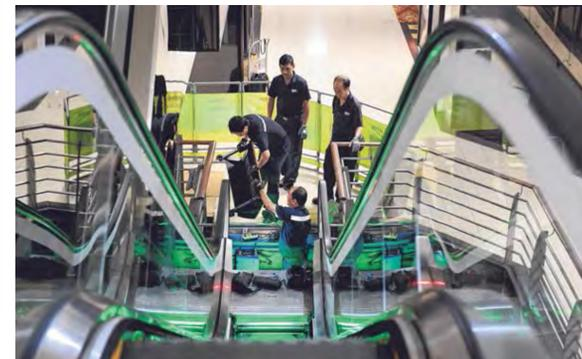
Once a month, Otis technicians descend on Fortune Centre before dawn breaks to do a routine check on the escalators. The floor plate is removed and steps are dismantled. Handrails and safety switches are inspected, while moving parts are lubricated (below). If all is in order, the parts are reassembled in time to turn the escalators on for the morning crowd.
