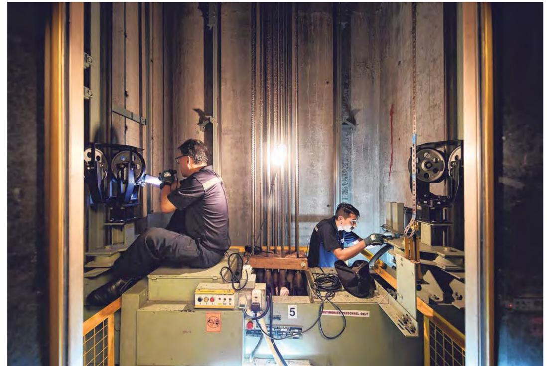
The next stage involves taking a ride on top of the lift car as they check various moving parts. As the lift travels from floor to floor, they inspect the door sensors and rollers, while making sure that no debris has accumulated in the door sill. The door was left open for this photo to be taken; lift doors are normally closed during maintenance work, for safety reasons.
