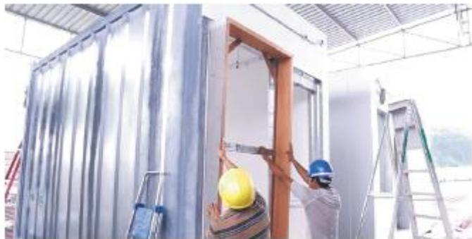
2. Modules arrive in Singapore's ports and are transferred to fit-out yards. Modules have to be fitted out within 1-2 weeks with lights, electrical wiring, sprinkler pipes, switches, fans, toilet piping, hot water supply, toilet floor casting and tiling, doors etc. Only the water closets and basins are left incomplete.
