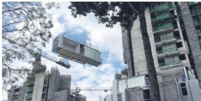
3. Every day, about 6-8 modules are delivered to the construction site to be lifted and assembled. Only after they are hoisted up are the sanitary drainage pipes connected manually to the units below them until everything is linked to the main drainage vertical stack. Mechanical and electrical services and floor tiling are then installed along the corridors to complete the project.
