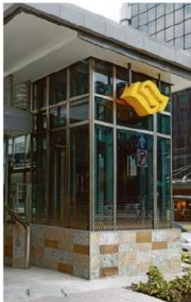
Bencoolen MRT Station is the deepest MRT station in Singapore at 43m below ground. PHOTO: SATO KOGYO
